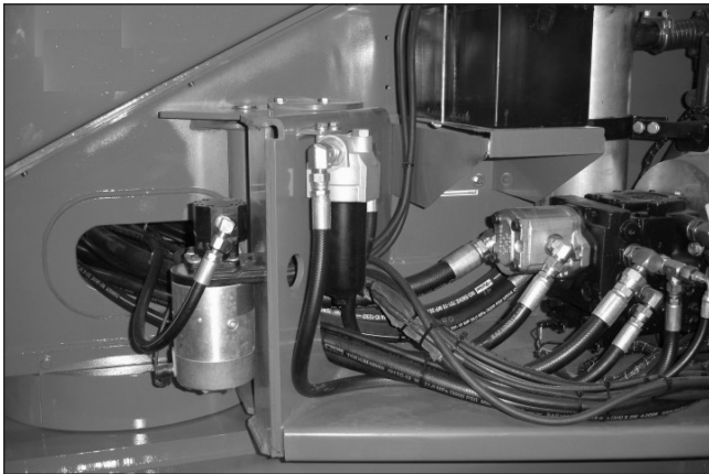
Figure 7.6 – Hoses, Tubes, and Fittings
