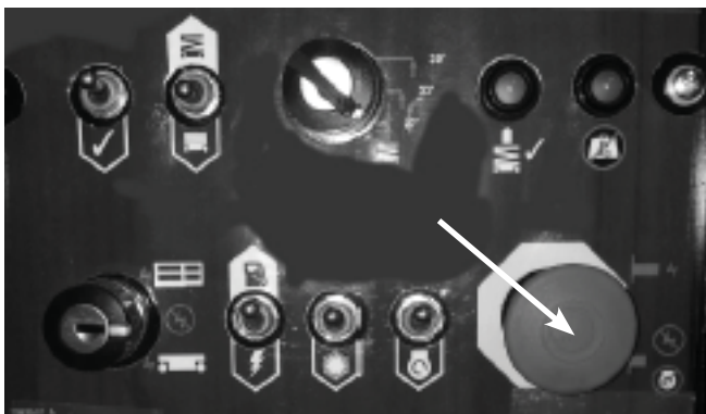
Figure 9.2 - Ground Control Box Emergency Stop Switch
